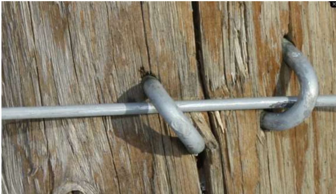
Staple balance: eleven o' clock and one o' clock.
