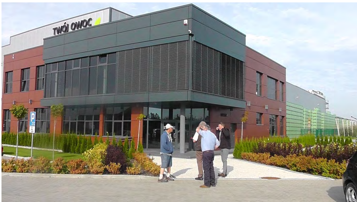
New cooperative packing facilities – 75% EU & Poland subsidies
